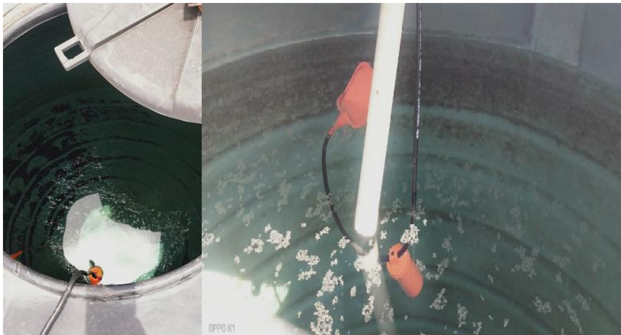
Figure 1: High level and Low level Cut-off Switch
