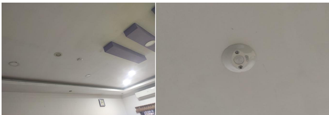
Figure 2: Room Sensors for lights and fans
