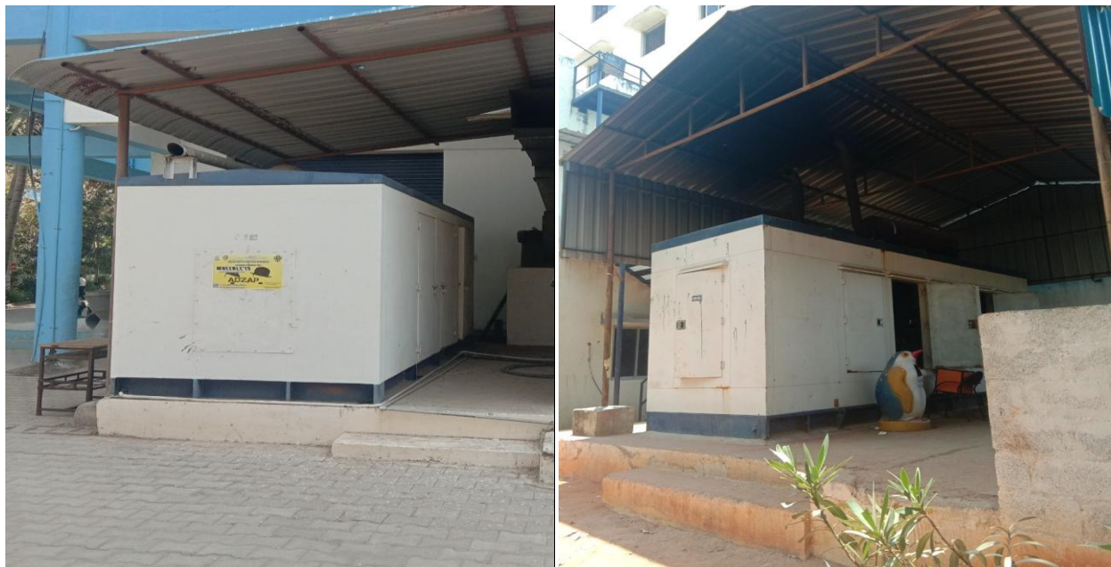
Figure 5: Gensets of capacity 500 and 600 kVA
