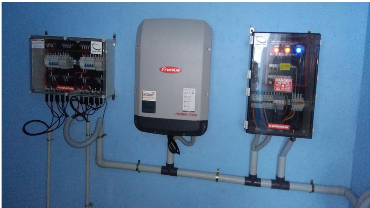
Figure 8: 20kW Solar Power Plant-2 Inverter Setup
