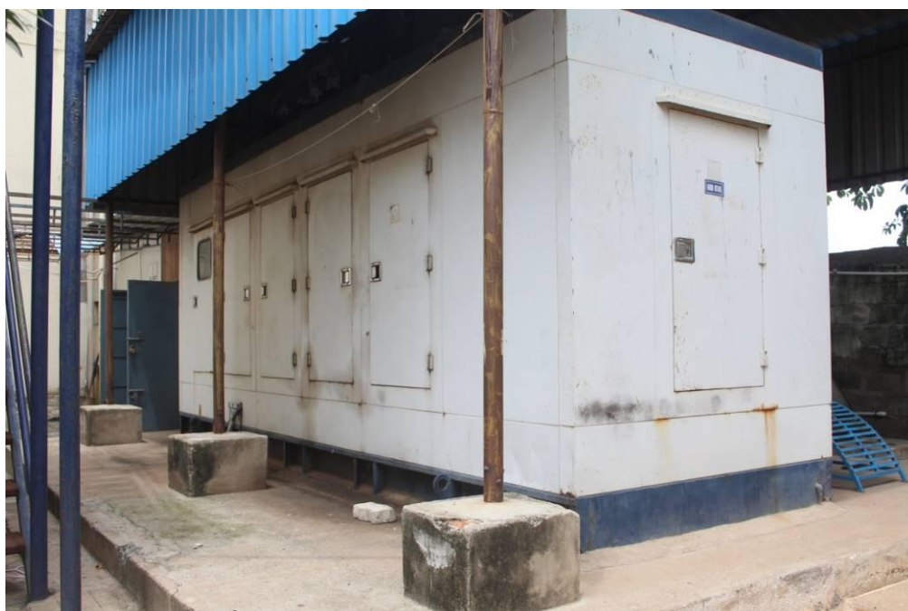
Figure 3: Gensets of capacity 500 and 600 kVA
