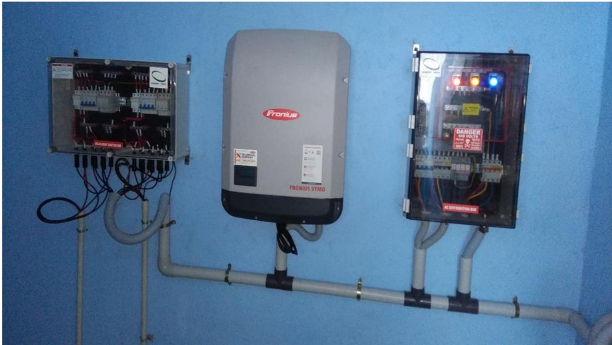
Figure 7: 20kW Solar Power Plant-2 Inverter Setup
