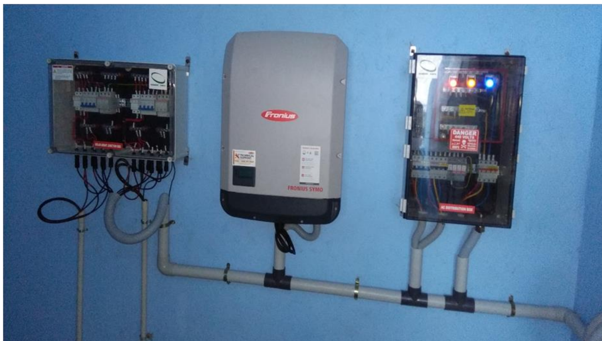
Figure 7: 20kW Solar Power Plant-2 Inverter Setup
