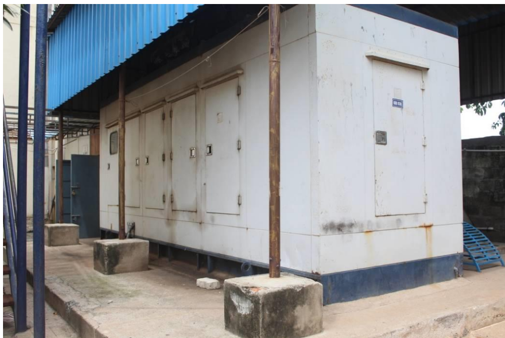
Figure 3: Gensets of capacity 500 and 600 kVA
