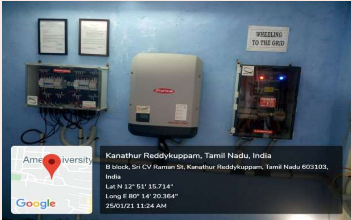
20kW Solar Power Plant-2 Inverter Setup
