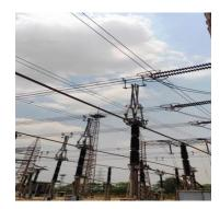
The 230kV yard uses gang operated double break isolator and the 400kV uses pantograph and Centre break isolator.
