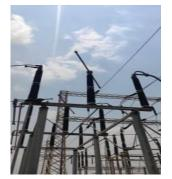
3. **Pantograph:** A pantograph mechanism is employed to make, break contacts
