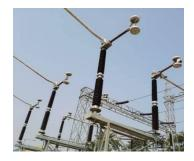
2. **Double break**: A central insulator of three insulator mounted on a post has the rotating male part and the other are mounted with 2 female contacts. When actuated, the male part rotates and makes contacts, hence closing the isolator. Since there are 2 break point, this is called as a double break isolator.
